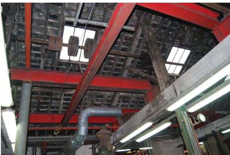
Plate 49. Remains of belt drives in the erecting shed
