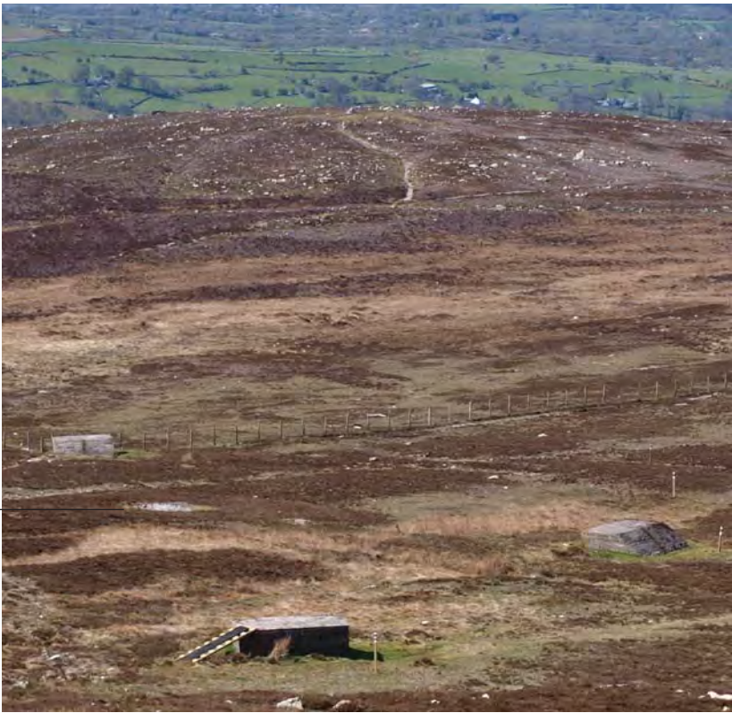
Plate 1. View of Cefndu Transmitter Station (PRN 887), showing mast base PRN 61279 surrounded by stay anchors
