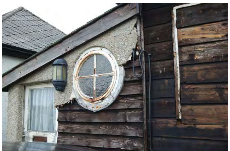
Plate 21. The original circular window at No. 7, Marconi Bungalows, and part of a blocked window
