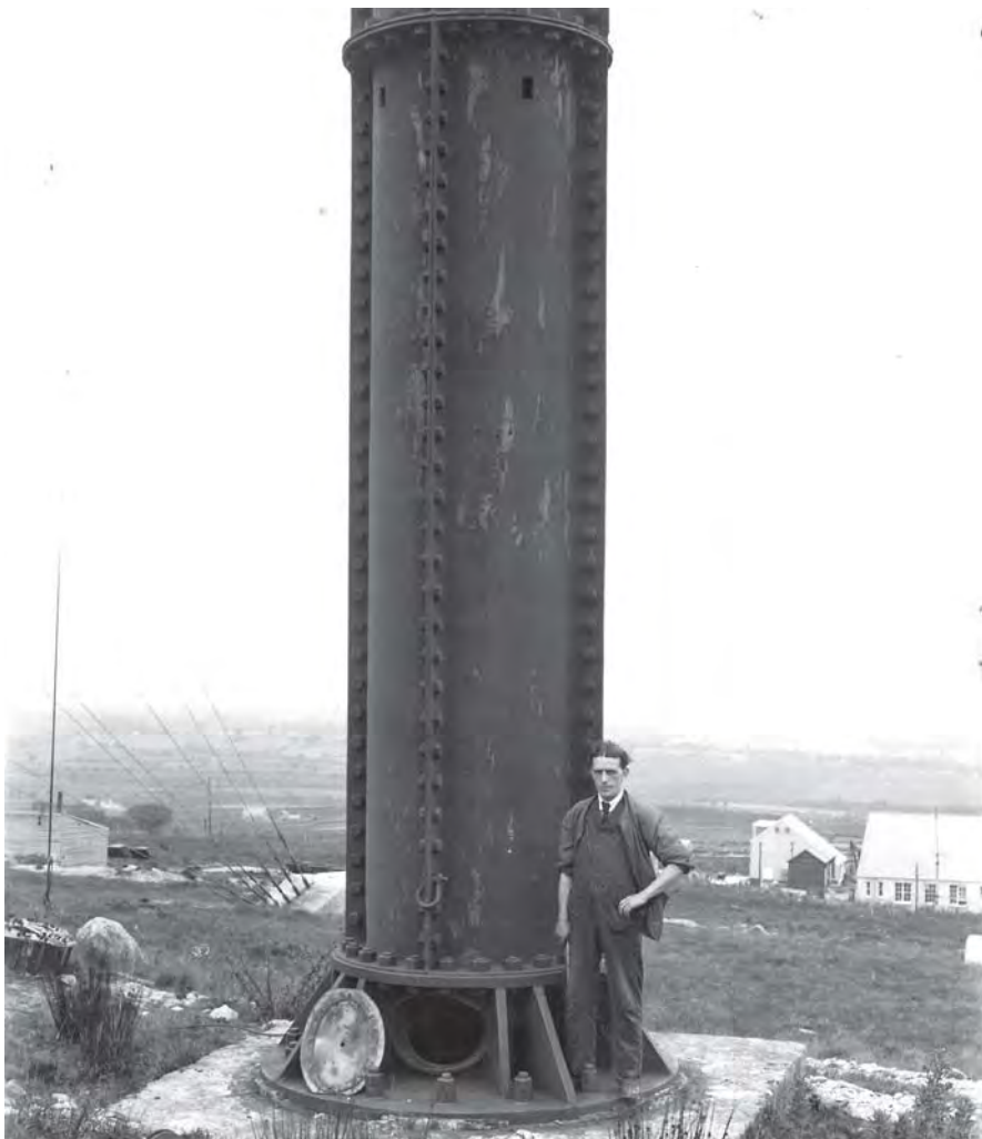
Plate 4. Base of mast, note open access hatch for maintenance and stay anchor to the left. Photograph dated 1912 but probably actually 1914 (The Marconi Company Ltd)
